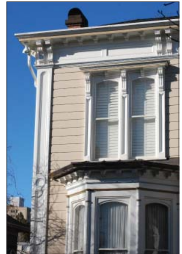
The fine Classical details help to define the facade and fenestration of this Italianate style.
