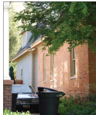
This recent addition reflects the design traditions of the original with a change in material to siding. The change from original to new is emphasized by a break in the wall plane and roof plane.
