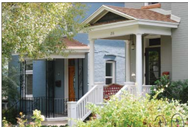
Wood columns and balustrades were commonly replaced with thin “wrought iron” railings and posts in the 1950s. This compromised the proportions and architectural integrity of the house.
