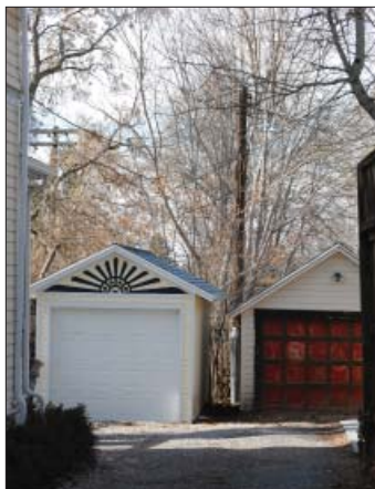
Continuing scale and/or use of early rear garage structures with shared access driveway.
