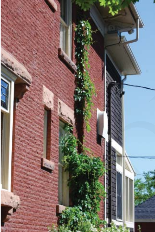
A rear addition which is subordinate to the house and differentiated by height, materials, fenestration and simpler profiles and details.
