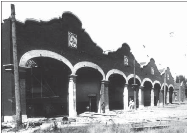
Trolley Square under construction.
