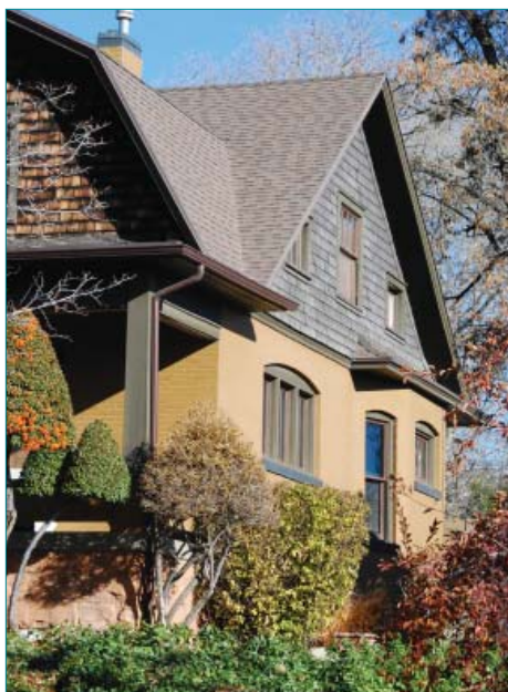
A considered color scheme here complements both building and setting.
