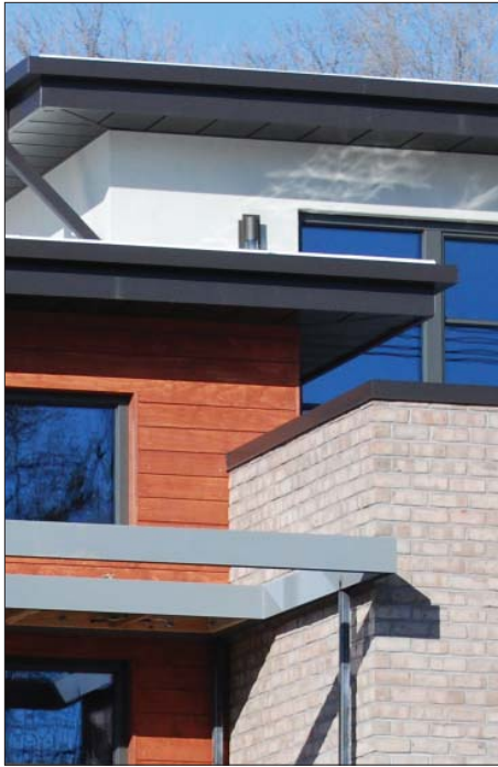
An interplay of several characteristic materials (brick, siding & stucco) and colors can help to integrate simple rectilinear forms with the palette of materials and colors of the context.
