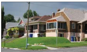
Enclosing a front porch will significantly compromise the architectural integrity of the house.
