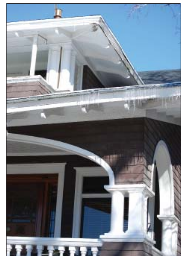
The deep eaves, rafter tails, arches and columns help to define the individuality of this bungalow design.
