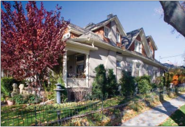
The creative use of dormers provides significant additional space in a way that complements the design of the house.
