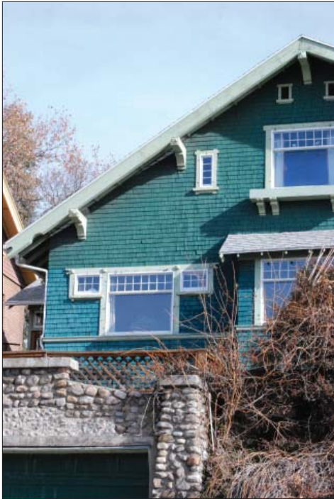
Early street facing 'sunken' garage using river rock facing.
