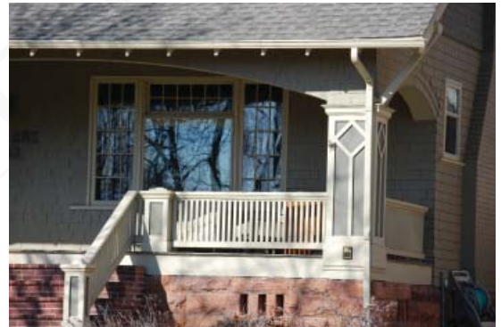
A rich palette of building materials, patterns and textures characterize individual buildings and the neighborhood as a whole.
