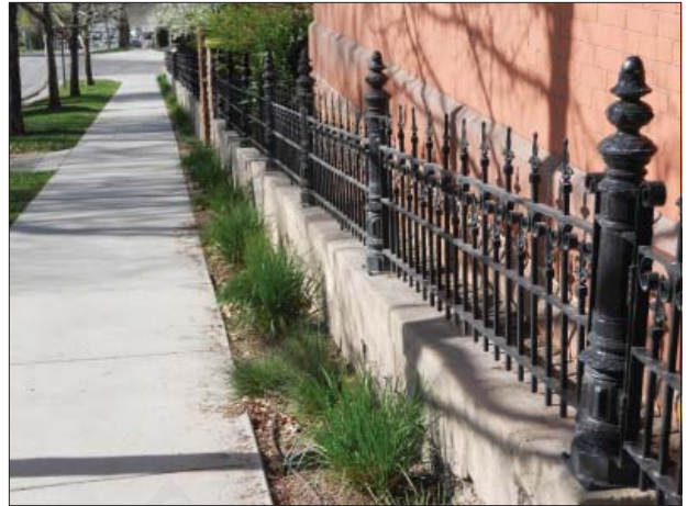
The low retaining wall supporting an ornate historic iron fence contributes significantly to the character of the streetscene.
