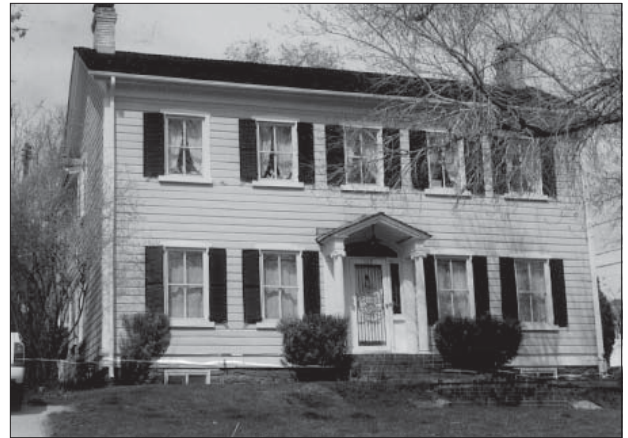
Classical Porch, at central entry.
