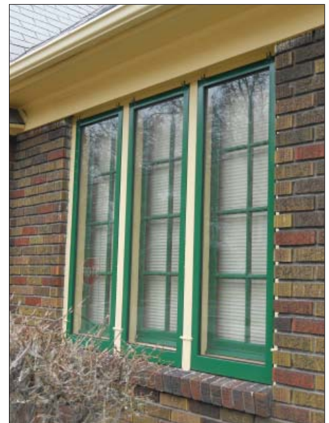
External wood framed storm windows designed to fit the primary framework of the original.
