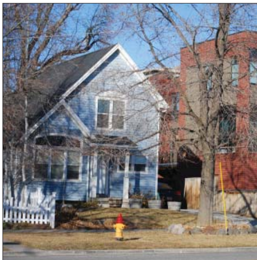
The solid to void ratio here closely reflects that characteristic of the setting and the historic neighborhood.
