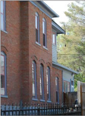
Rear addition which reflects the eaves heights and profiles.
