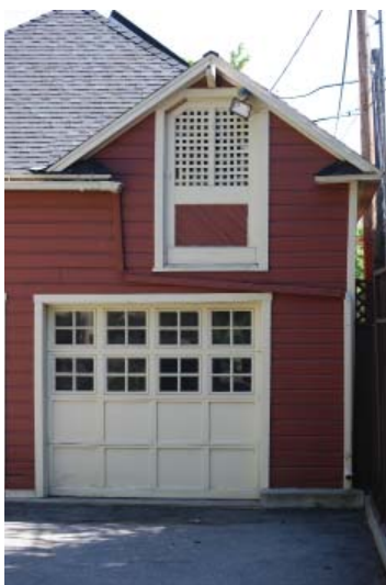
Carriage house with hay loft door
