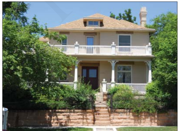
The form, construction, detailing and materials of a retaining wall may complement both the architectural setting and character of the neighborhood.
