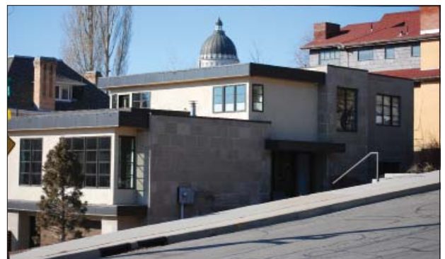
The width of this building reflects building width and scale in this setting, while the strong horizontal emphasis of one street frontage is counter-balanced by the vertical emphasis of the modules of the other frontage.
