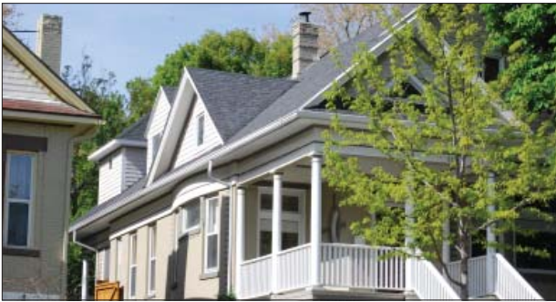
Rear addition designed to integrate with the historic roof form.
