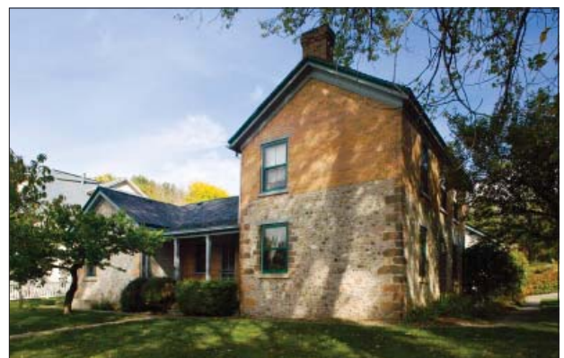
The addition here takes the form of a new single story wing to the left of the two story earlier building, itself with an early addition of the second floor.
