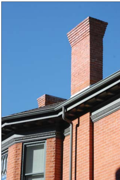
Variation in the brick texture and the pointing profile are used in this case to define the wall, the window bay and the chimneys.
