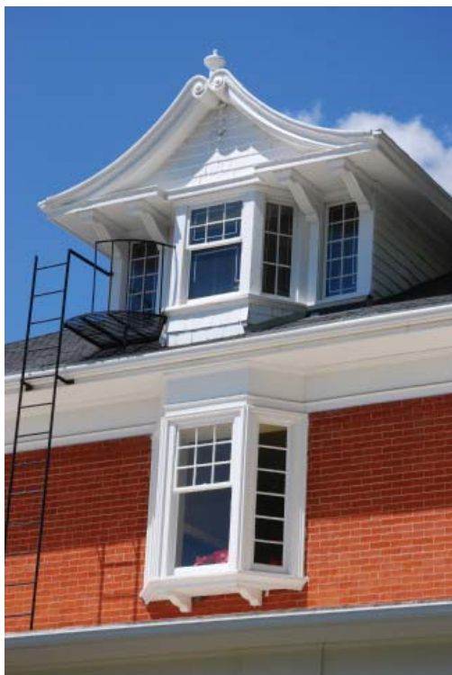
Finely detailed brickwork warrants special care in maintenance or repair.
