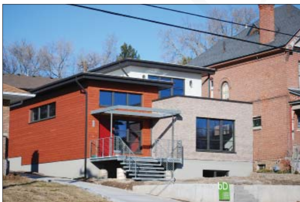
The massing of this building is designed to mediate between adjacent single story and two story buildings, increasing in height incrementally as it steps back from the street frontage.
