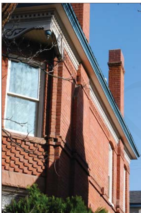
Brickwork lends itself to an endless variety of creative architectural compositions with associated decorative relief and textures.
