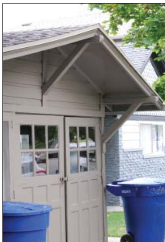
Street facing accessory structure reflecting the house design, and using a pair of side-hinged doors.
