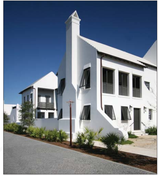
Much of the design composition of these buildings relies upon the fenestration pattern 'punched' into sheer white walls, strong gables and soaring chimney.
