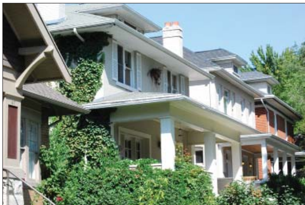
Square columns in various designs create detailed variety and a visual richness in this complementary series of full-width porches.
