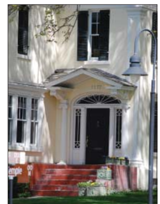
The doorway, the proportions of opening and framework, sidelights and transom/fan lights, porch hood, decorative details, and the design of the door itself, combine to celebrate the entrance.
