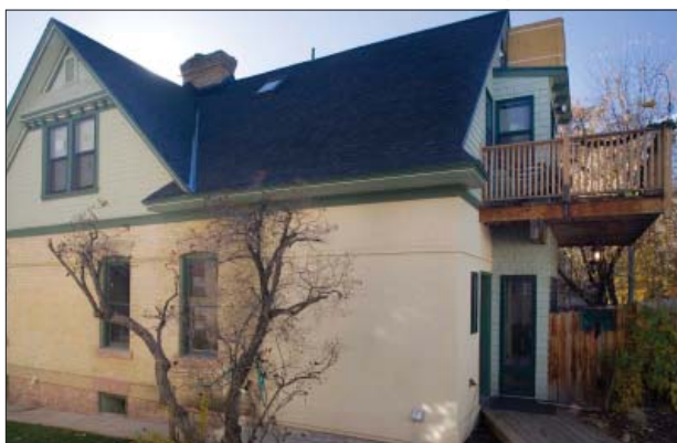
This rear addition continues the design tradition and language of the original with a change in external materials.
