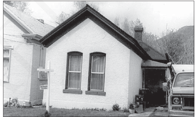
This is an unusual example of a front facing Greek Revival style building in the Capitol Hill Historic District. Despite the rarity of its orientation, its massing, stucco finish, pronounced wood cornices and fascia are clearly in keeping with this style and period.
