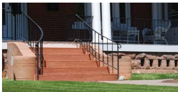
Local sandstone is widely used in a variety of ways, making significant use of form, texture and decorative detailing.
