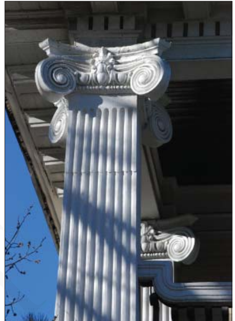
Periodic maintenance of painted surfaces maintains weather resistance and enhances the character of the building.
