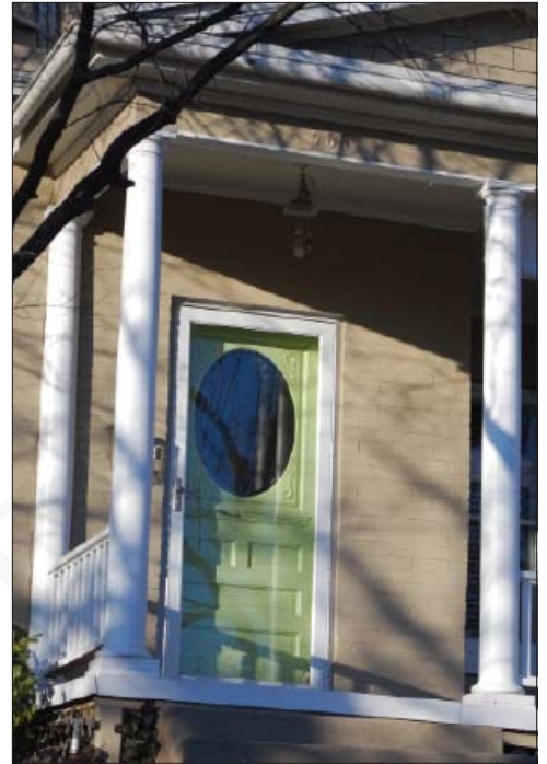
A storm door designed to enable the form and detail of the door to be readily seen.
