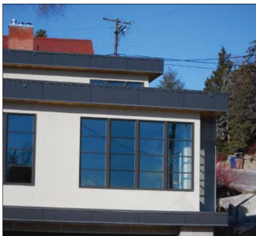
Despite the contrasting geometric modules of this building, the subdivision of the fenestration helps to convey a sense of human scale and to integrate the design with setting.
