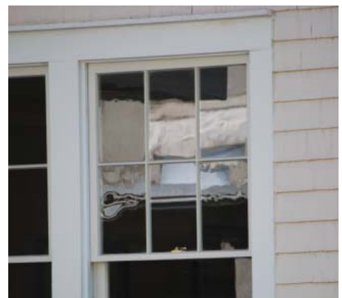
The difference between the characteristics of early glass is seen in contrast here adjacent to the more recent glass in the replaced center light.
