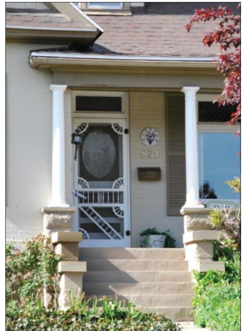
In this case the storm door and screen provide a decorative addition to the original design of the door, although some original detail is obscured.
