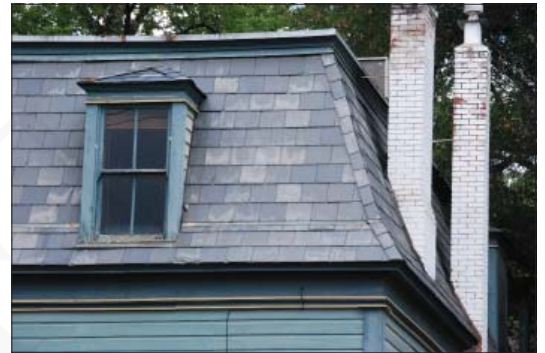
Natural slate is rare in the city and is the most durable of traditional roof materials, usually requiring only piecemeal replacement of damaged individual slates.
