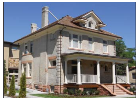
The Stanley F. Taylor building, a residence dating to c. 1906 was recently seismically upgraded as part of an extensive rehabilitation.
