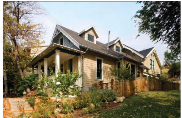
The rear addition steps back from the side facade of the house and integrates two story living space in a manner which does not dominate the original building.
