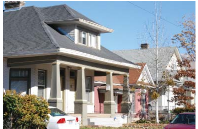
Orienting the entry to the street is preferred. Establishing a "progression" of entry elements, including a walkway, landscaped elements and porch also is encouraged.
