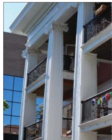
Multi-family and apartment buildings reflect the development of the area.
