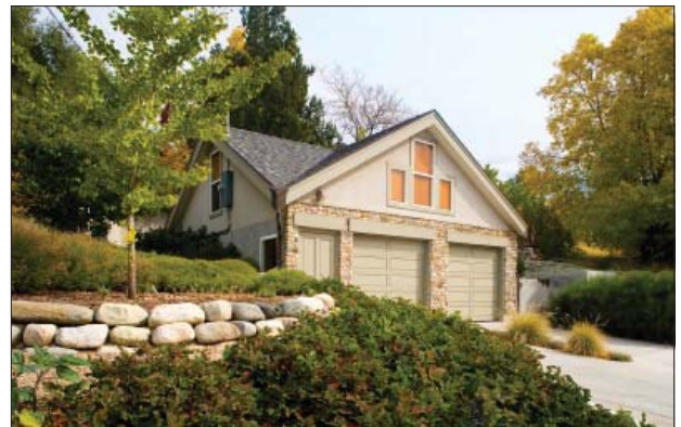
Recent garage with living space above designed to reflect scale and character of the context.
